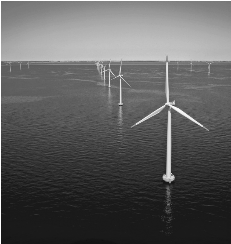
FIGURE 9.15 Nysted wind farm in Baltic Sea, Denmark. (Photo courtesy of Siemens.)
