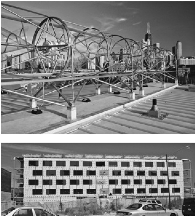
FIGURE 9.5 Eight helical horizontal axis wind turbines, 1 kW each, on top of building. (Photos courtesy of Kurt Holtz, Lucid Dream Productions.)
