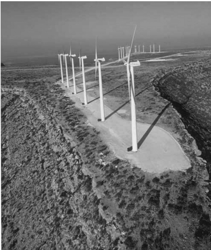
FIGURE 9.13 Wind farm on Southwest Mesa, near McCamey, Texas. Example of mesa with one row. (Photo courtesy of Cielo Wind Power.)
