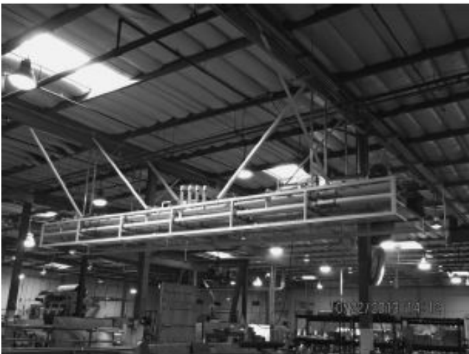
FIGURE CS6.2 Sophisticated multi-service modules prefabricated
