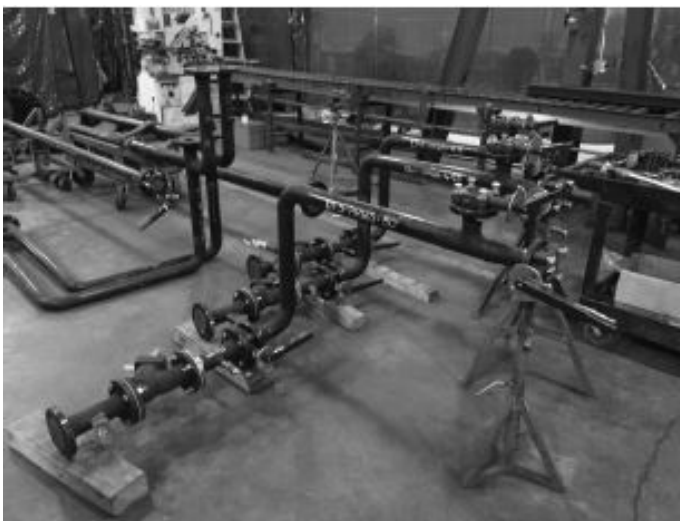
FIGURE CS6.1 Complex prefabricates enabled by BIM
