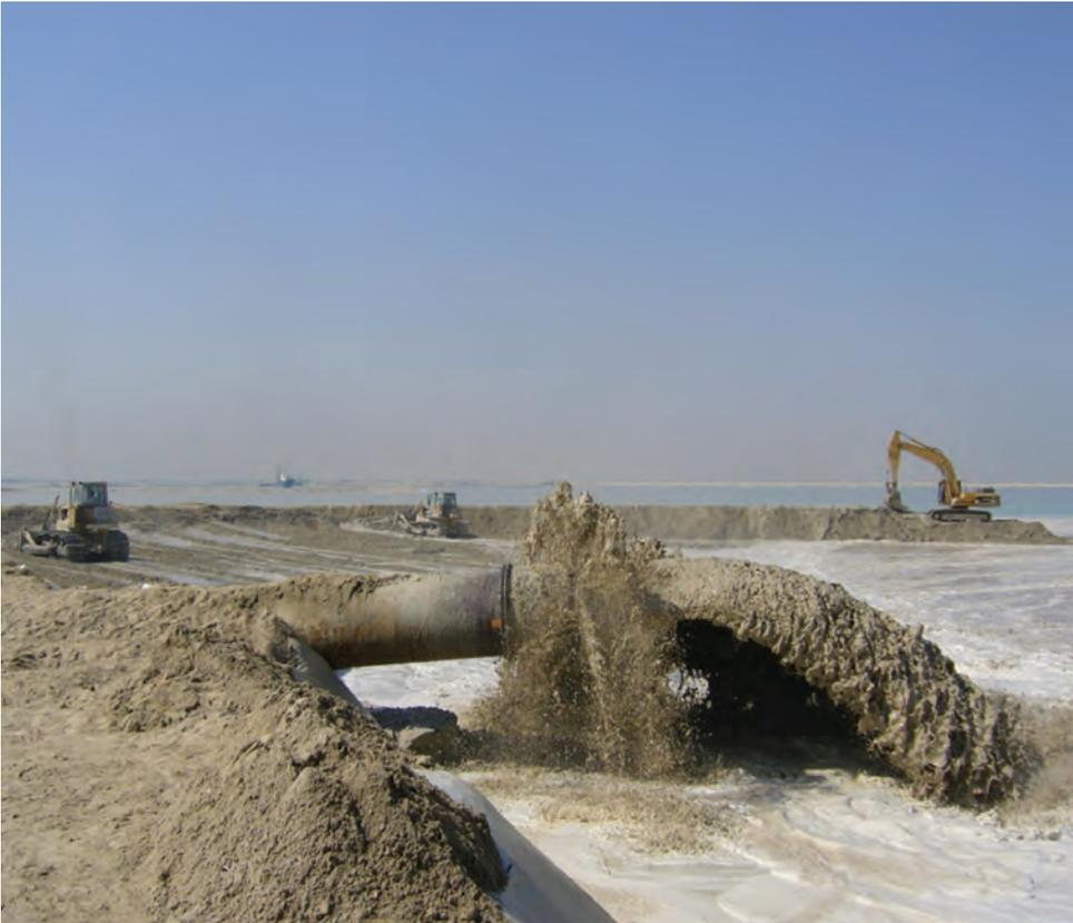
with certain technical measures and under certain conditions, cohesive and fine-grained materials (clay, silt) also may be used. The use of carbonate sands is also highlighted.
